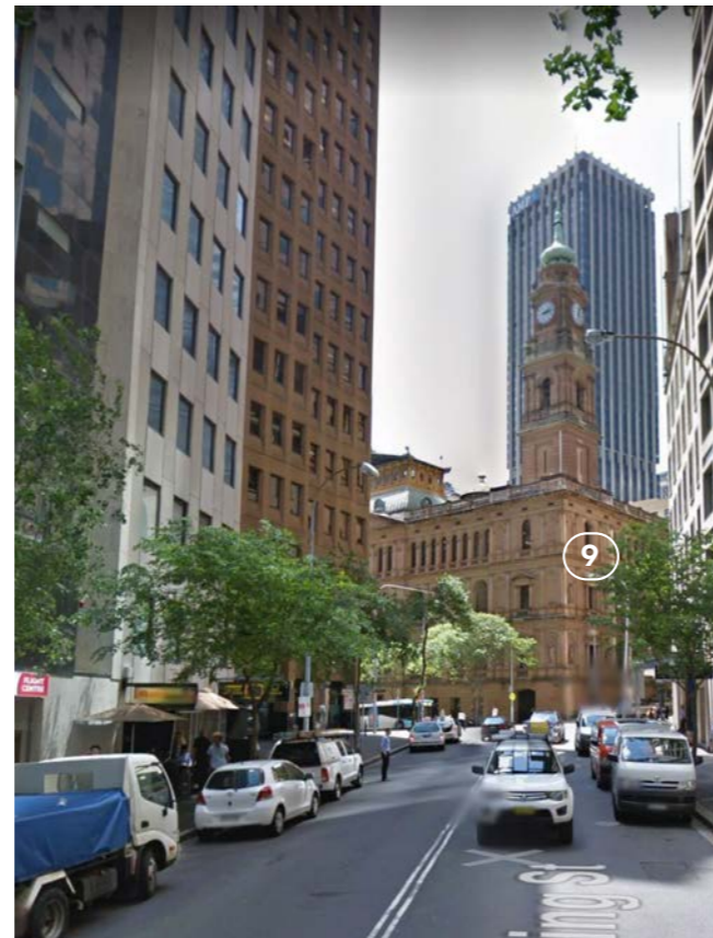
Department of Lands Building from Spring St.
