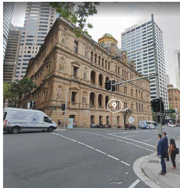
Former Department of Lands from Loftus St.
